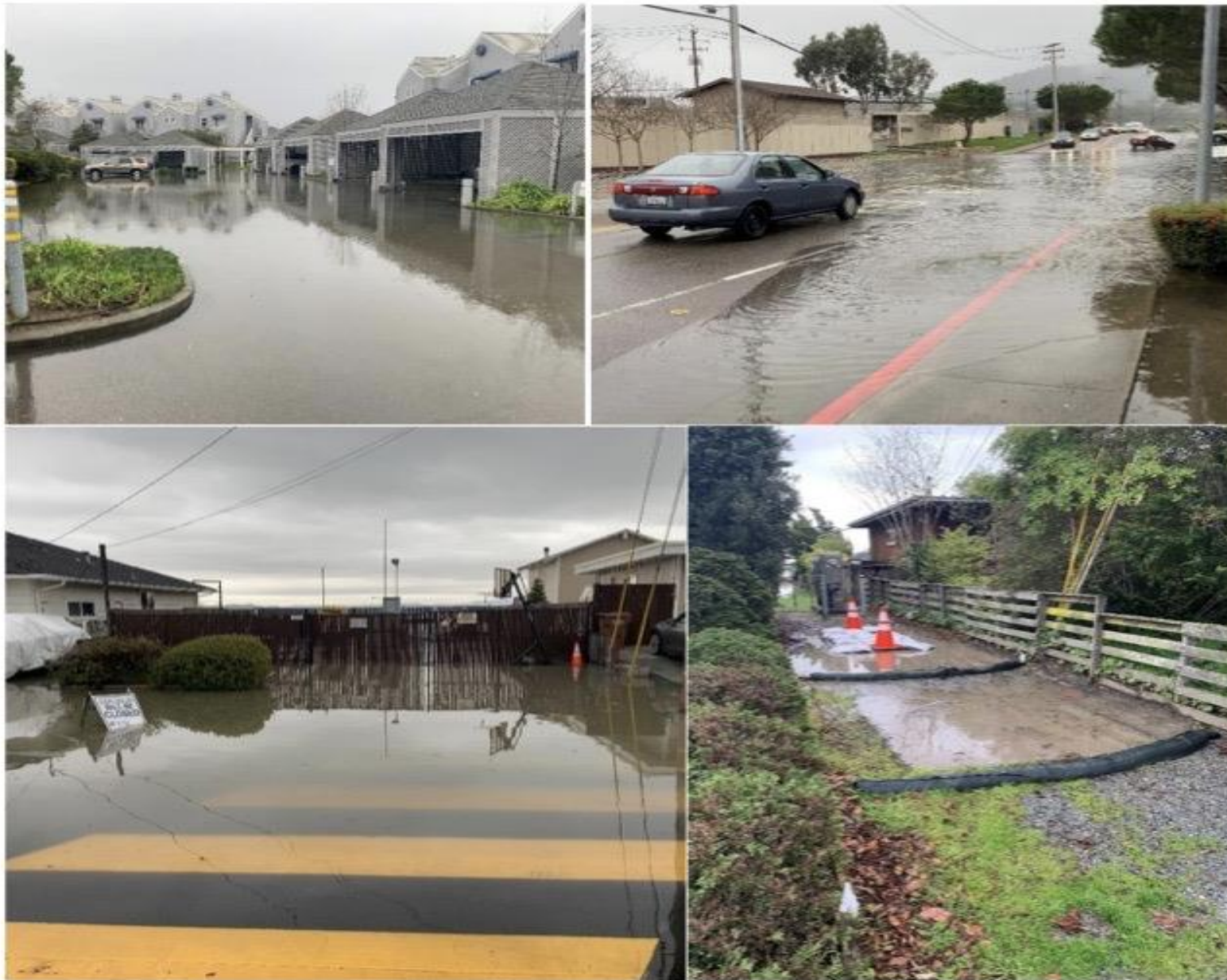
Figure 2-4: Standing Water During a January 3, 2022 King Tide Event near Lucky Drive (Top) and Along Golden Hind Passage at Ebbtide at Sanitary and Stormwater Pump Stations (Bottom)
